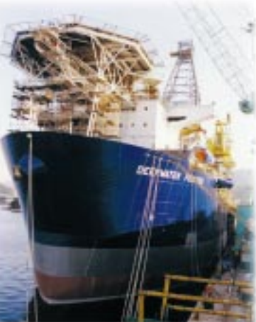
Designed for service in waters up to 10,000 ft deep, DEEPWATER PATHFINDER is the first of a four ship series of 56,000gt dynamically positioned, deepwater drill ships building to ABS class at Samsung.
