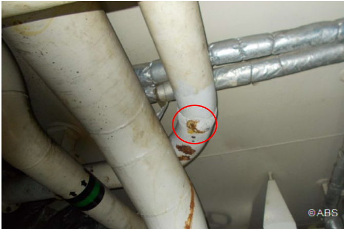
Ballast pipe repaired with patch
