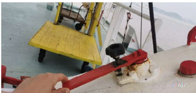
Rescue boat winch speed engaging lever inoperable
