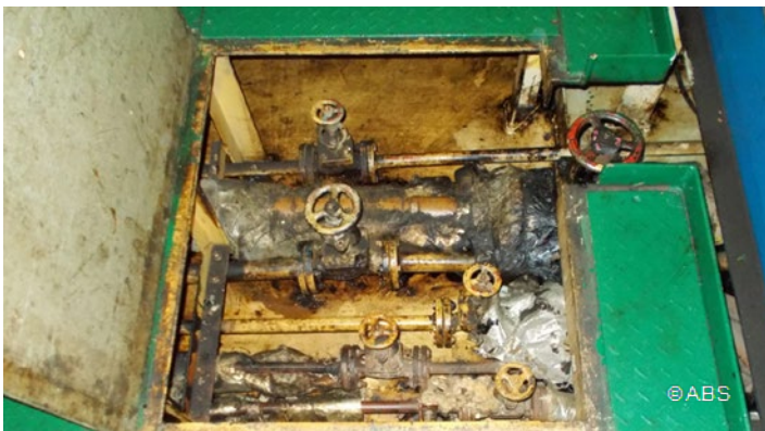
Purifier room fuel oil piping insulation missing
