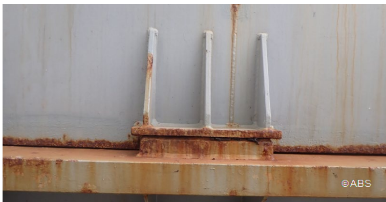
Cargo hold hatch cover is touching metal to metal instead of resting on the pad, due to worn out pad material
