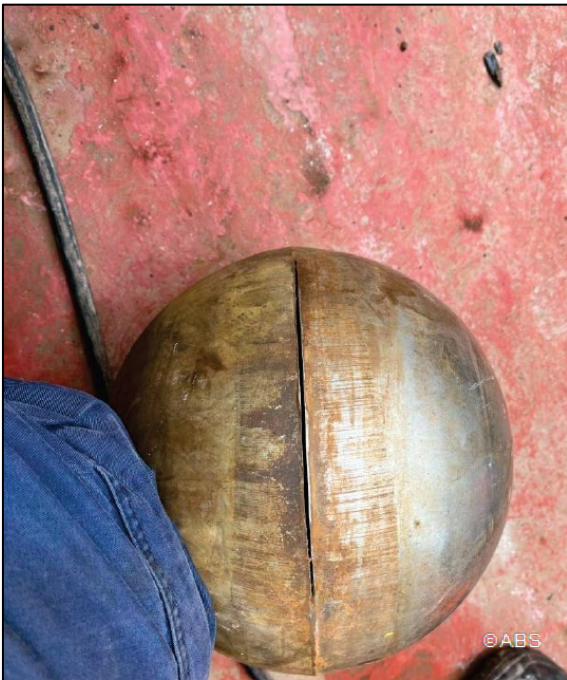
Tank vent head floater damage
